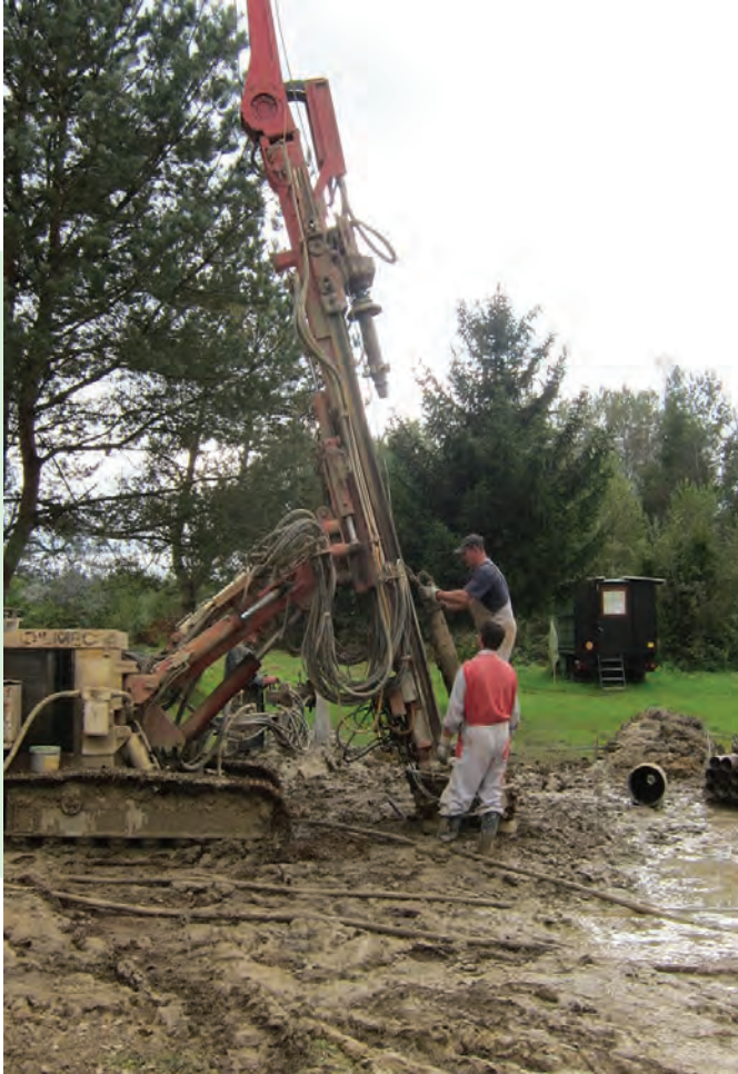
Drilling to a depth of 20 m for the installation of pilots for the foundation at Prilozje
