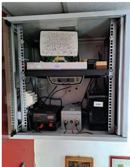
Layout of devices in the cabinet of the Črnomelj permanent GNSS station
