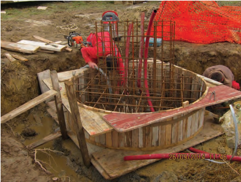
Concreting the foundation and pillar at Prilozje
