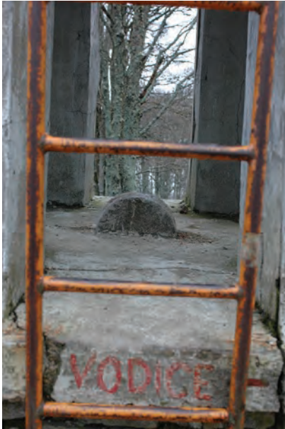
The lower reference point of the first-order trigonometric point Trdinov vrh today (left) and its appearance when it was erected in 1934 (right)
