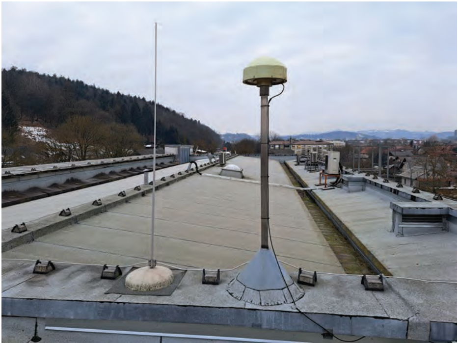
Antenna of the Ljubljana permanent GNSS station
