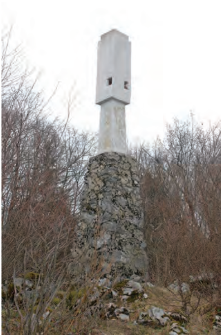
First-order trigonometric pillar at Debeli vrh
