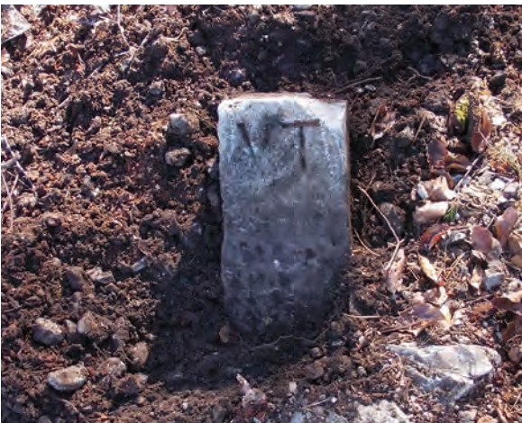
Loza (876 m): third-order trigonometric mark no. 160 in the trigonometric district of Postojna.
