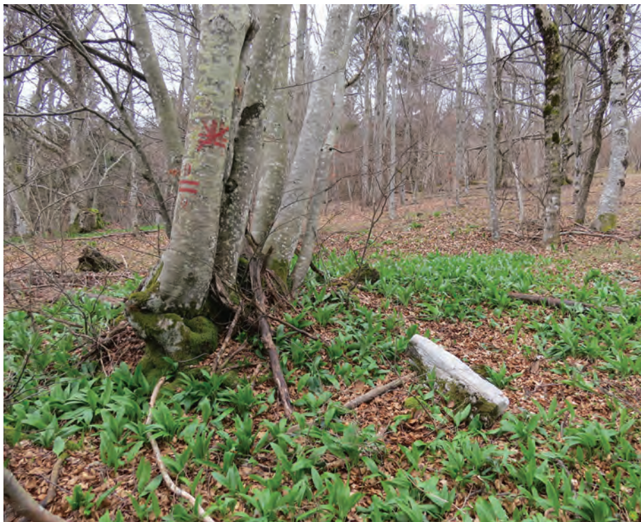
The uprooted boundary mark of the tripoint of the cadastral municipalities of Selšček, Cerknica and Grahovo.
