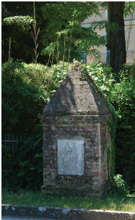
Jesolo, Italy: a Venetian boundary brick pillar from 1791. The total height is 2.4 m and the cross-section at the base is 80 cm × 80 cm.
