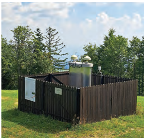
View of the point AREH where continuous GNSS measurements are carried out (below) and details from the project documentation (above).
